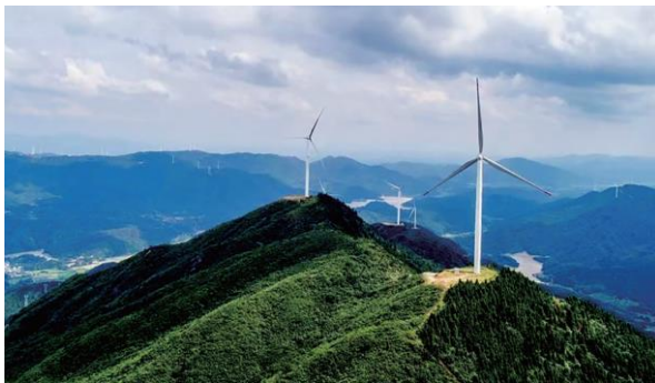
Wind Power Project in Moorabool, Australia
